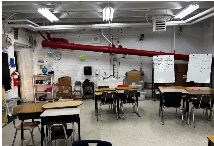
Existing Classroom Conditions
